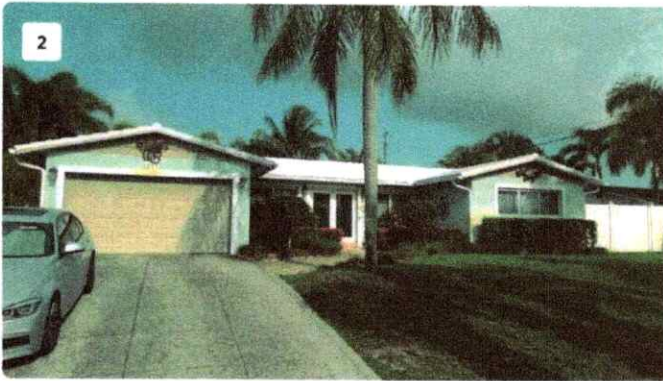
Project: Rigg Chang Date: Jun 6, 2025, 9:05 AM Creator: Frankie Fernandez
