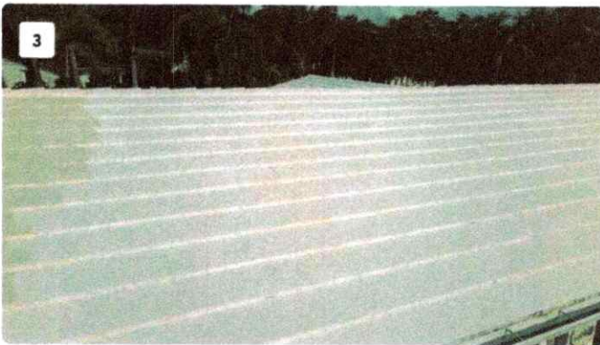
Project: Rigg Chang Date: Jun 6, 2025, 9:20 AM Creator: Frankie Fernandez
